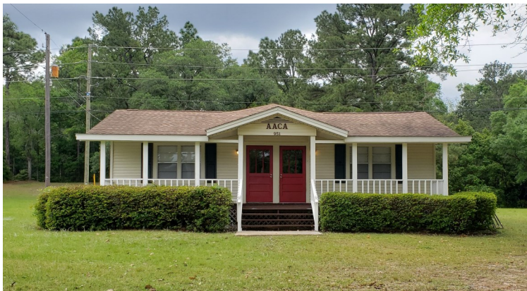
AACA Deep South Region Club House.
