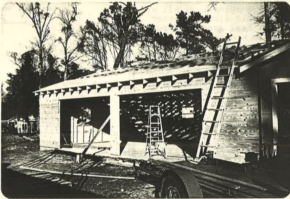
BILL & JEANIE DOBBS' NEW ANTIQUE CAR GARAGE UNDER CONSTRUCTION.
