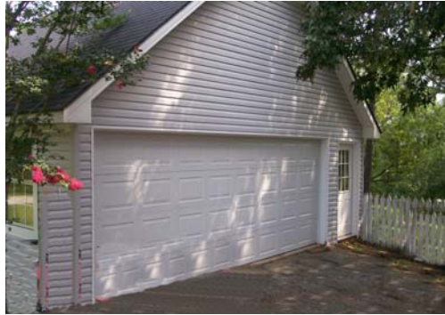
We installed the standard roll-up door plus the essential walk-thru door.
